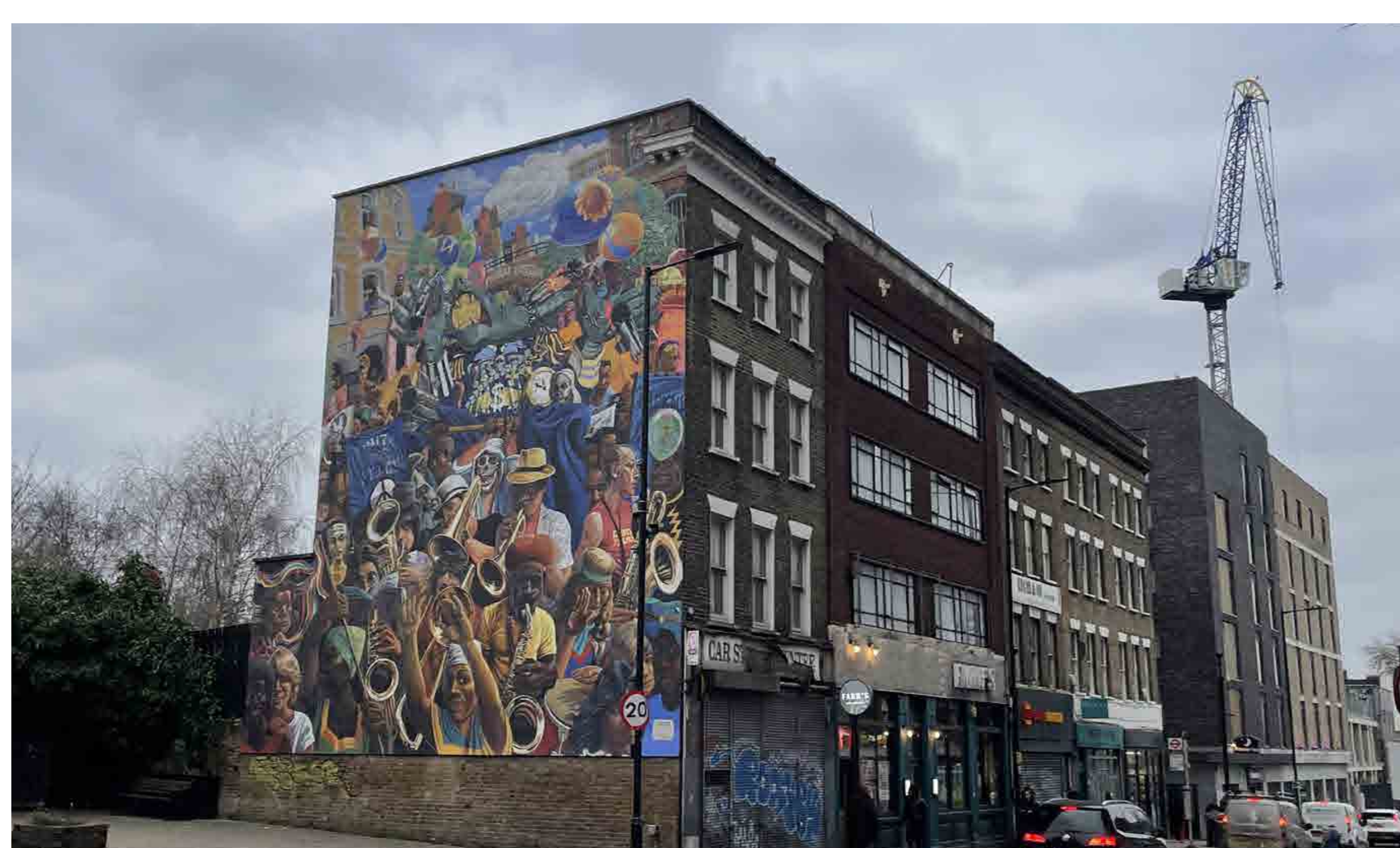
Side view and front of the existing buildings
